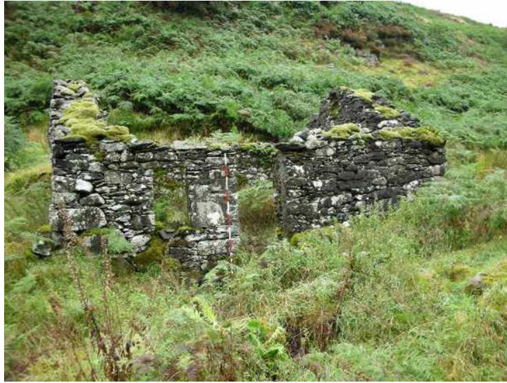
Structure B looking west
