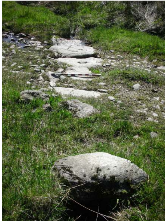
Site 30 Track and Culvert
